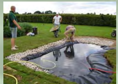
Building an eco pond in the UK
